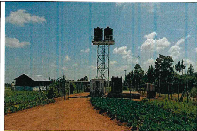
Borehole, water harvesting & storage in Laikipia
