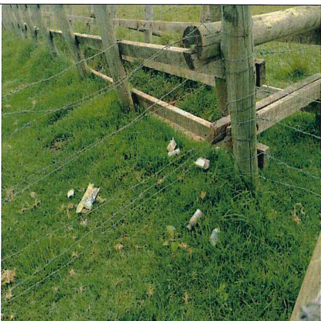
Solar Powered electric fence in Narok
